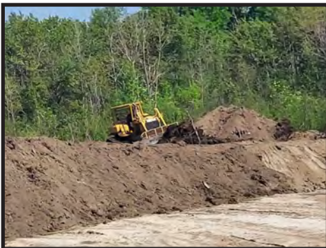
Building Berms for Pistol & Archery Ranges
